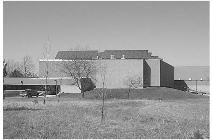
Warm water for the Phoenix Sports Center pool at UW-Green Bay is provided by the Solar Mining Company, Wisconsin's first solar utility (see page 4).
