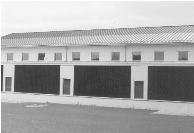
This 2,300 square foot Solarwall® pre-heats ventilation air for Mary Ann Cofrin Hall, a classroom building of the University of Wisconsin-Green Bay.
