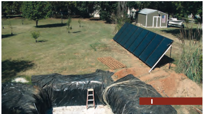
H, I - The authors recycled the solar panel shipping pallets to build a 4- by 4-foot room on top of the heatstore bed for the solar appliance and pipe manifolds. The week of Oct. 12, the authors measured 145°F (63°C) at 3 to 5 feet deep. The system's solar panel array was producing a maximum water temperature between 168°F and 178°F (76°C and 81°C) on days the sun shined. They were ready to fill the hole and put the heatstore in observation mode.
